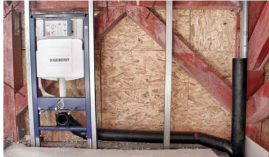
Whether commercial clerks, mechanics or plastics technicians – Geberit apprentices show their plumbing skills during the social project in Romania.
