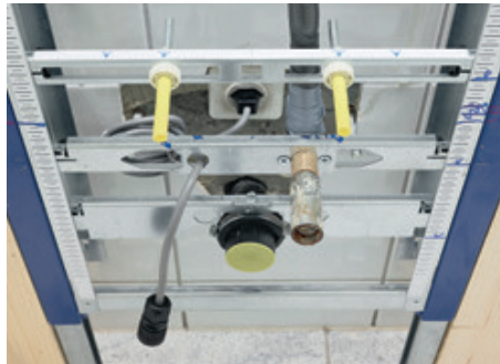
↑ The Geberit Duofix installation elements for urinal systems are prepared for the installation of the models Preda and Selva.
