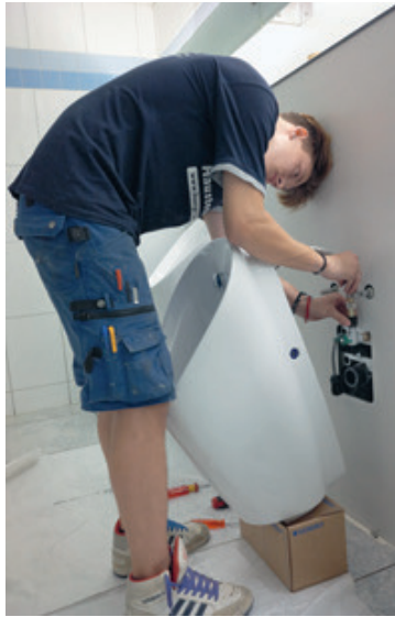
↑ Because the reinforced braided hoses have been specially prepared at the factory, connecting a Geberit urinal to the water supply is taken care of in next to no time.
