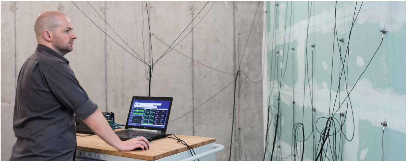
Samuel Pasteur, acoustics specialist at Geberit, measures the sound transmitted from a concealed installation to a neighbouring room using acceleration sensors.
