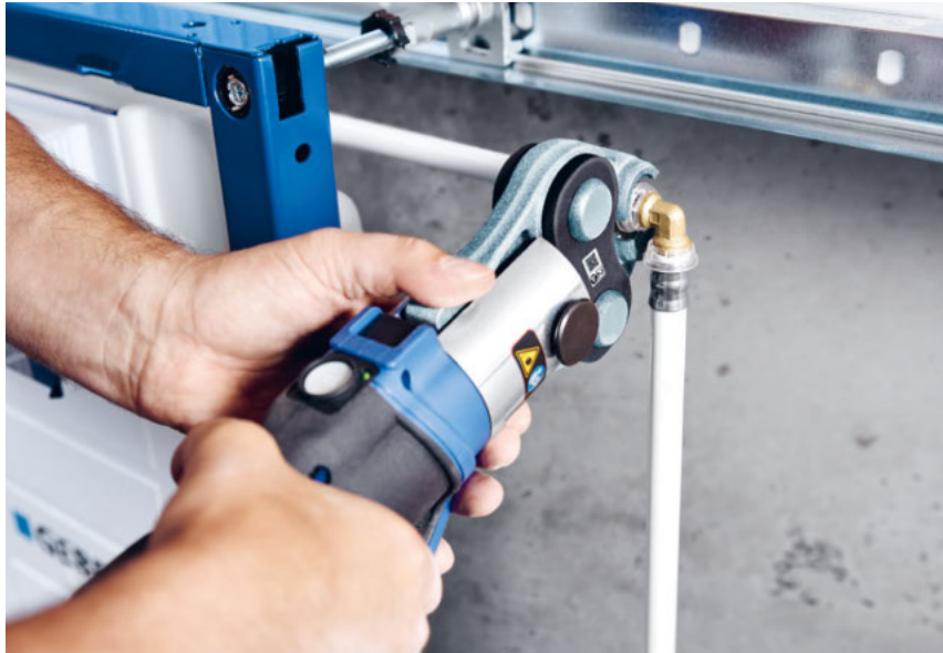
↑ The press connections are reliable and leakproof, and make it possible to work efficiently on the construction site.
