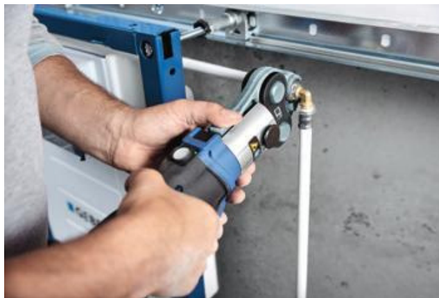
↑ Geberit pressing tools fit precisely to the profile of the fittings, thus ensuring faultless workmanship.
